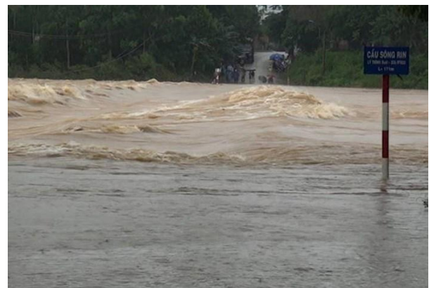
Fig. 3 Rin River Bridge fully inundated by the
