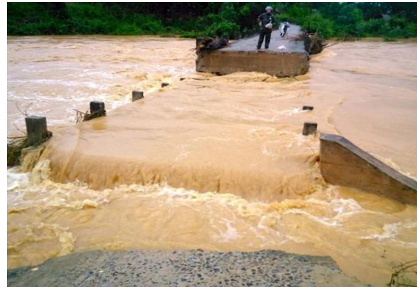
Fig. 2 A bridge collapsed in Thua Thien Hue province, Vietnam, 2016
