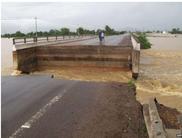
Fig. 1 Bridge in Binh Dinh was shattered by the flood, 2013
